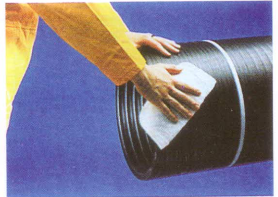
Make sure that spigot end, socket and sealing are clean from sand, moisture, dust etc.
