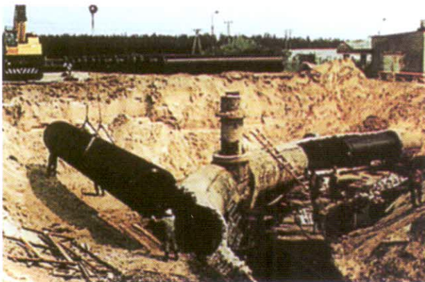
Swiecie, Poland; Relining of 650 m, 1800 mm corroded concrete pipe with Ø 1500 mm Spiro pipe. Total project completed in 8 weeks.
