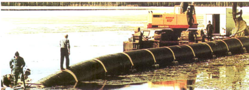
Swiecie, Poland; Relining of 650 m, 1800 mm corroded concrete pipe with Ø 1500 mm Spiro pipe. Total project completed in 8 weeks.
