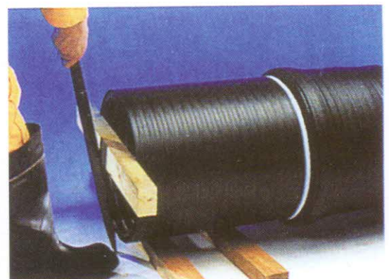
Place spigot end against the socket opening, making sure the pipes are still aligned. Gently push the spigot into the socket using suitable force until the stop-mark is at the socket opening. Use a plate or plank to avoid damage to the spigot or socket. Larger dimensions can be put together using an excavator. Be sure to protect the socket opening with a sheet or plank.
