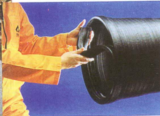
Install the rubber sealing into the groove.
