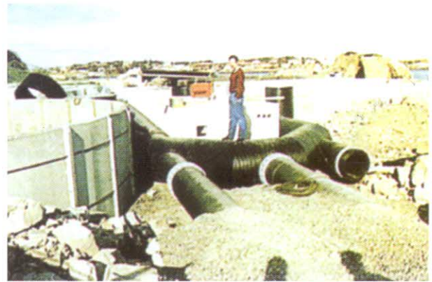
Averø, Norway; Weholite Spiro used in a fish farm. Diameters from 600 mm to 2000 mm ID.
