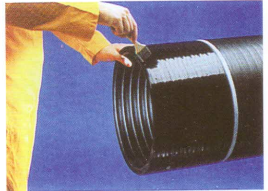
Apply lubricant evenly onto the spigot end.
