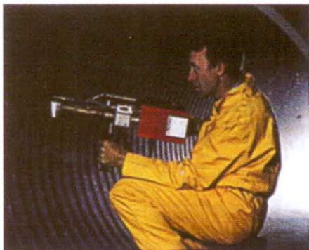
Hand extrusion welding
